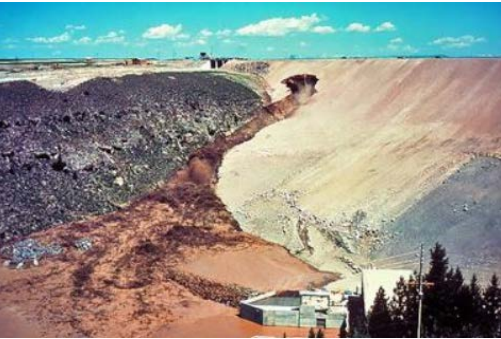
Beginning of the dam failure
